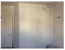
and remove sanding dust with vacuum or damp cloth. If after the initial mist coat, additional plaster is necessary, it will once again need to completely dry before reapplication of a second mist coat. Applying a non-reduced emulsion, will cause it to dry too quickly and will not properly adhere to the surface. Also, the use of a vinyl emulsion will form a skin on the plaster and may be prone to peeling as well as alkali issues.
