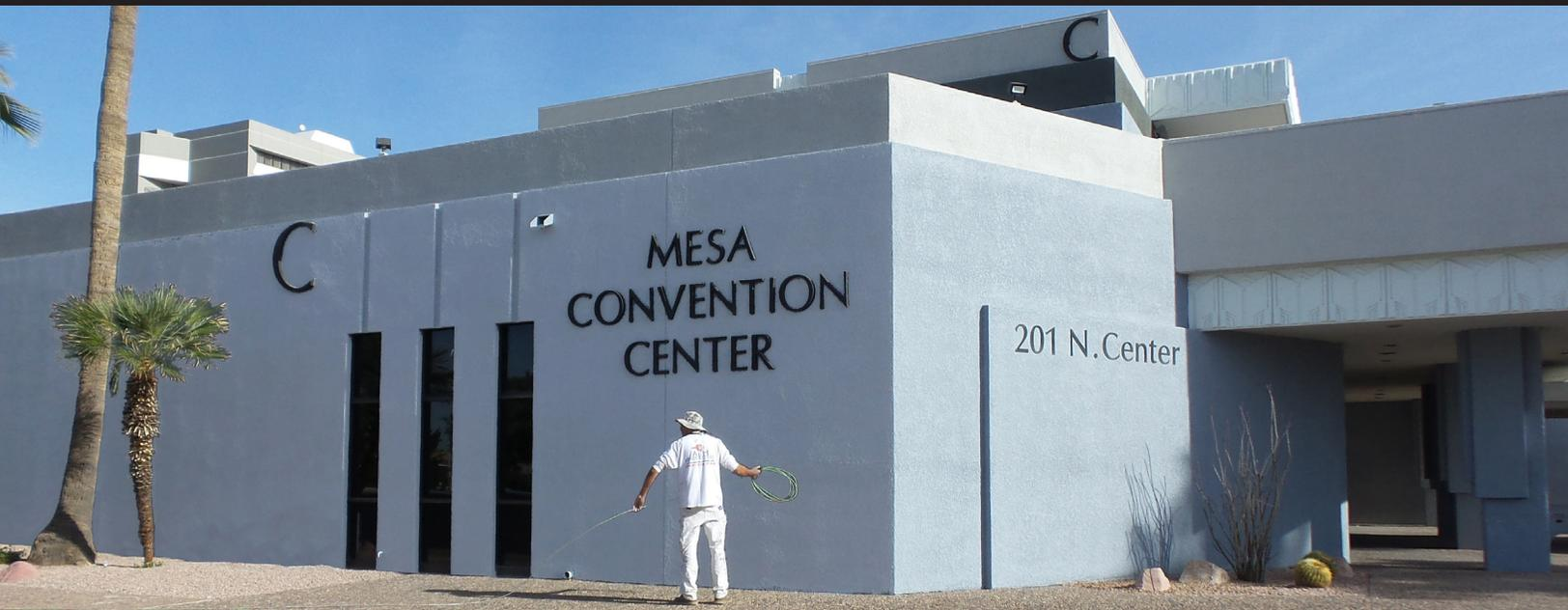
One recent project where that level of attention was key was the exterior repaint of the Mesa Convention Center and Amphitheatre. A variety of substrates across the properties called for a range of products including EFF-STOP Premium for priming masonry and Smooth BLOCFIL Select for priming block walls and planters—and ultra-premium paints: EVERSIELD for walls and stucco, and ARISTOSHIELD for metal railings, doors and fences.
