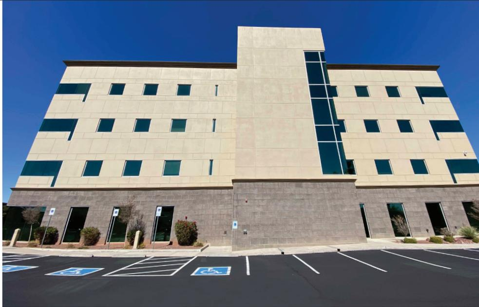
Finding the right primers was key as well. Vay's Dunn-Edwards rep suggested their FLEX-PRIME Select as a protective sealer with great bonding properties for the upper floors. The first floor of the building was built with concrete block veneer, a different type of substrate than the other three floors. It would require its own bonding patch coating, the Dunn-Edwards-sourced RAINGUARD Blok-Lok, used in many anti-graffiti applications.
