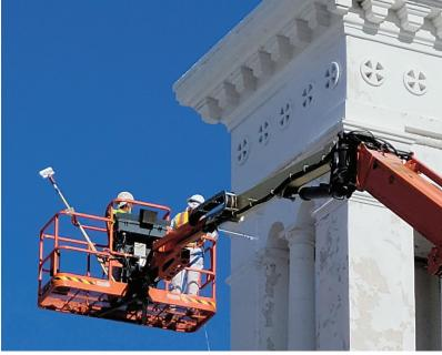
Determined to get the job done, Dougall estimated he needed a 150' boom lift, but a 185' lift was the only one available. The job required barricade permits from the city because the lift would occupy three lanes of an adjacent street. The city quickly complied, and Desert View's four-man crew persevered. They pressure washed and scraped the tower walls, applied two coats of a customformulated elastomeric primer, and then two coats of EVERSHIELD® Ultra-Premium Exterior Flat Paint in white.
